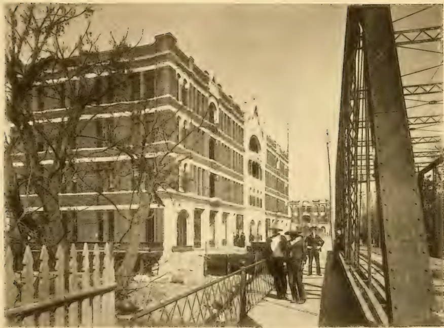
ALAMO FIRE INSURANCE BLD'G AND NAVARRO STREET BRIDGE.
